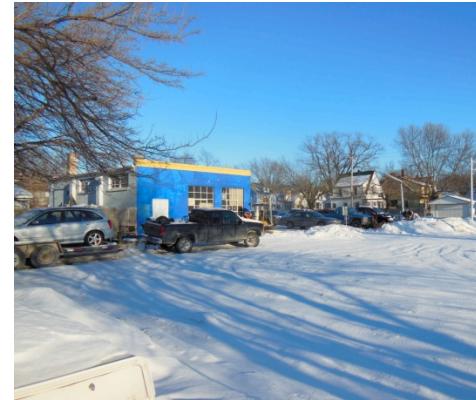
West side of the property, from vacant lot at 2040 E Johnson
